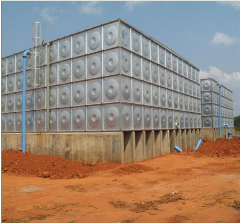
Water Tanks Installed at Lunyangwa, Mzuzu Water Supply
